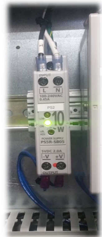
Figure 1 example of 5vdc power supply
